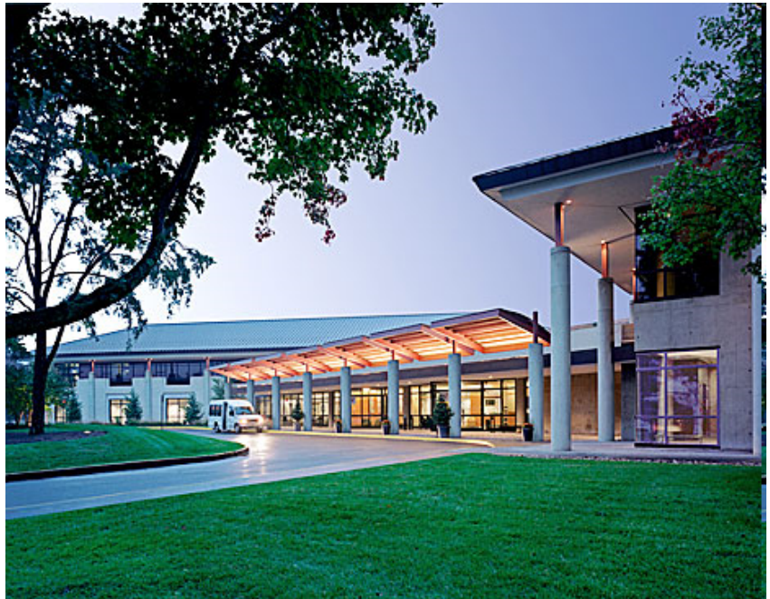
National Conference Center, Leesburg, VA
